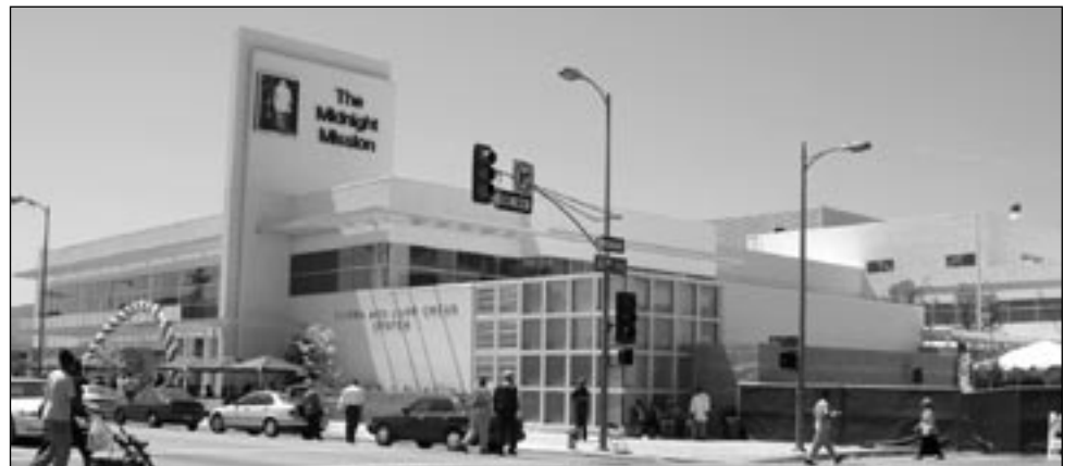
Demolition of the Caltrans building (left) created space for the new police headquarters. The Midnight Mission opened a long-awaited new facility.
